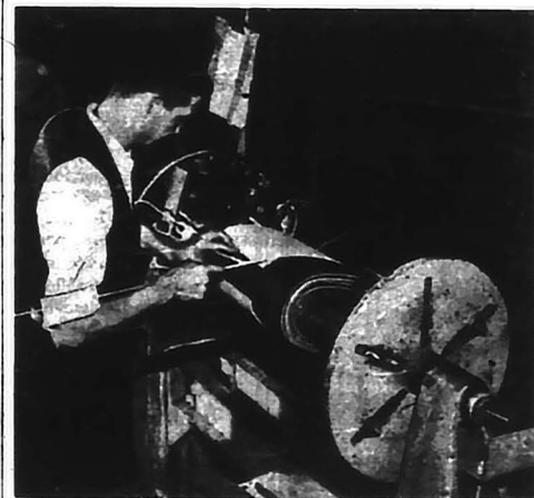
A delicate operation in transformer building is the winding of coils as demonstrated by this skilled Packard worker.
